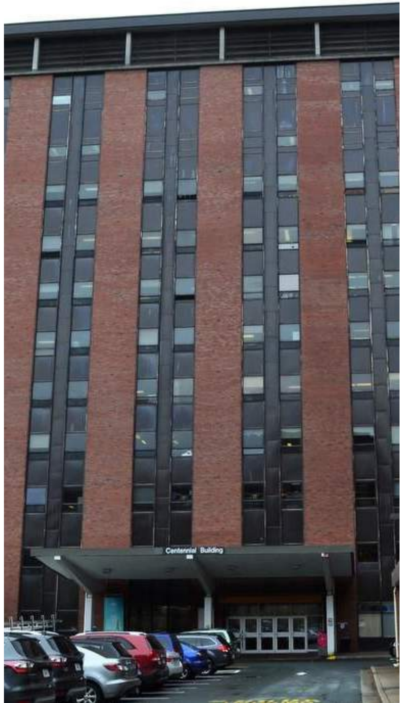
NOVA SCOTIA HEALTH AUTHORITY Centennial Building - QEII
